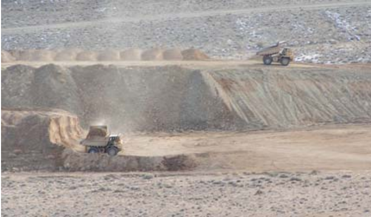
Reclamation activities at the MacArthur Mine waste rock dump
