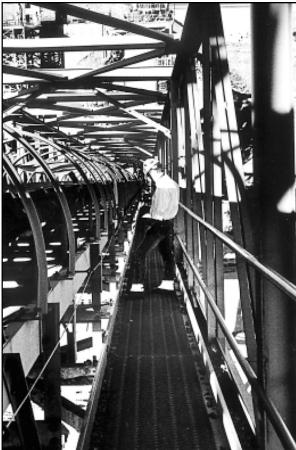
Safety specialist, Randy Squires, checks on equipment at the Newmont Mine East Carlin site
